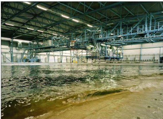
The new carriage of the Seakeeping and Manoeuvring Basin .
